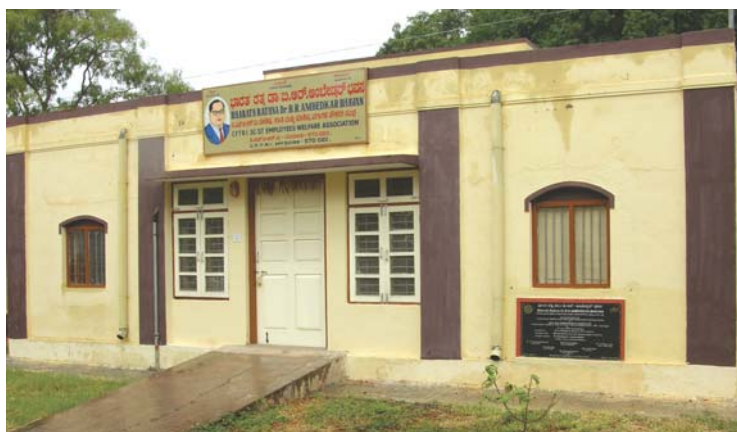
Frontal view of the CFTRI SC/ST Employees Welfare Association Building - Bharath Ratna Dr. B.R. Ambedkar Bhavan at CFTRI campus
